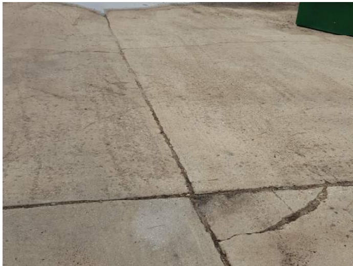
Photograph 7: Isolated low-severity scaling, low-severity corner break, loading dock, looking west.
