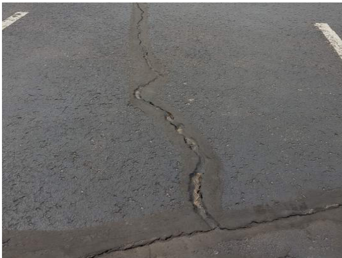
Photograph 15: sealed high-severity longitudinal and transverse cracking, south parking area, looking west.
