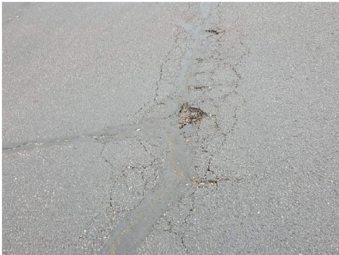
Photograph 11: low-severity fatigue cracking, isolated pot holes, and rutting, northeast parking area, looking north.
