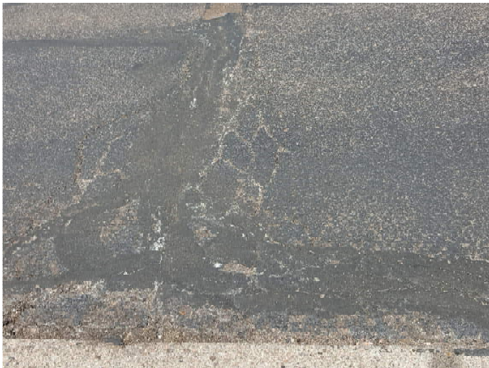
Photograph 3: Low- to moderate-severity fatigue cracking, NE entrance (Area No. 3), looking north.
