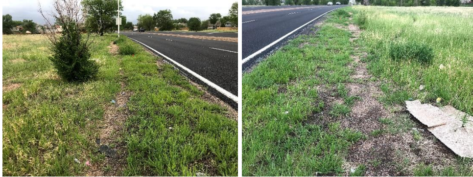
Figure 2. Lack of Sidewalks
