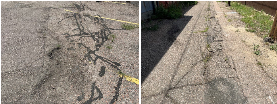
Figure 14. Deteriorated Pavement
